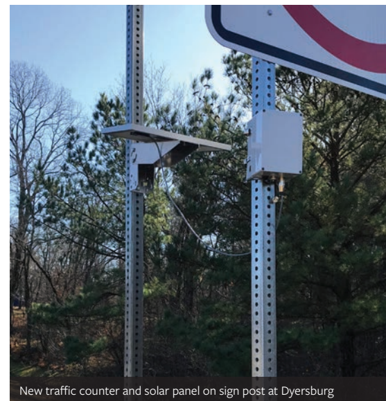
New traffic counter and solar panel on sign post at Dyersburg
